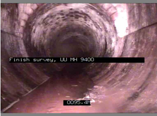
_3db50f29-7db9-4df9-83fd-ffc15a0464f2.jpg, 00:04:36, 95.40 m Finish survey, UU MH 9400
