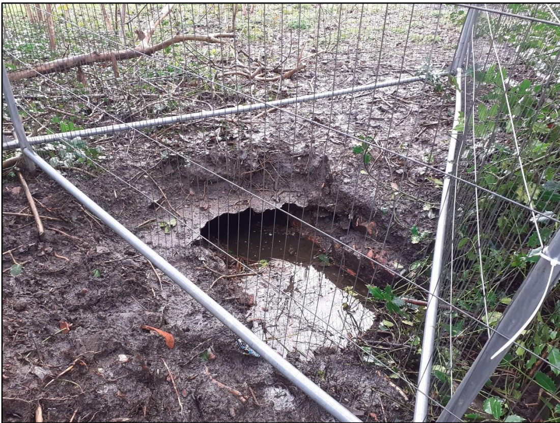
Figure 3.5: Culvert, Taken Facing West
