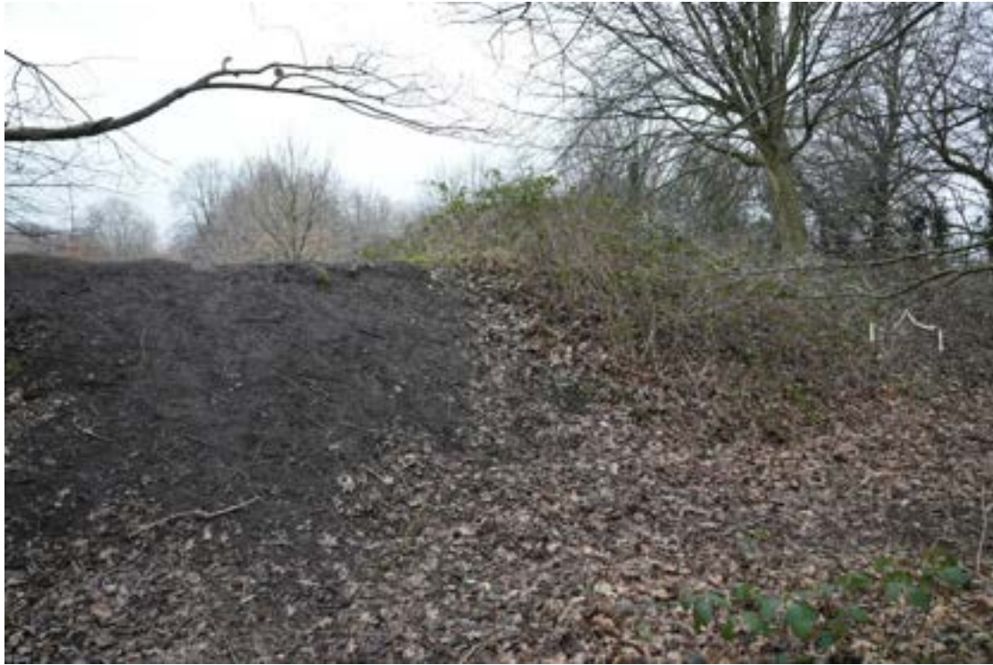
Photo 42: Image showing earth bank at TN10.
