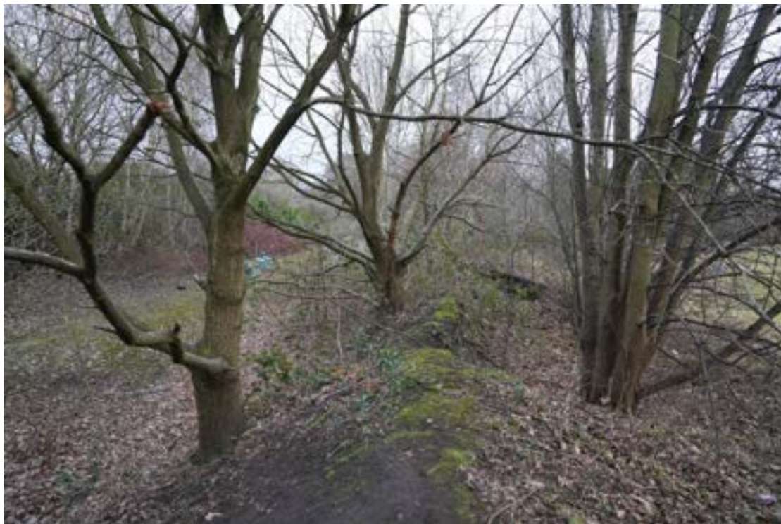
Photo 41: Image showing earth bank at TN10.
